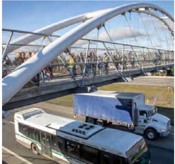
Pedestrian / bicyclist bridge over highway
