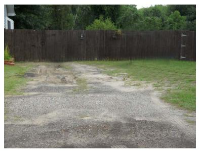
All surfaces shall be maintained. Concrete must be kept sealed and if cracks do develop they must be sealed to prevent moisture from causing further deterioration. Asphalt must also have cracks sealed and have the surface treated to minimize deterioration. Gravel must be graded and replenished on a regular basis.
